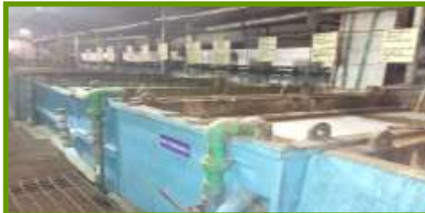
15 Tanks "Pretreatment Process" Which Optimized... Process Water Consumption LPG Gas Consumption Chemical Consumption a)Electricity Consumption
