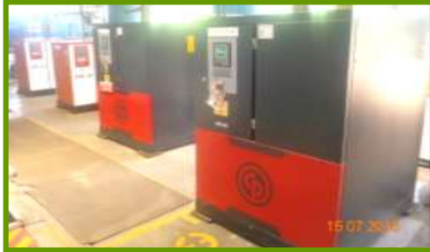
Optimized compressed air thru centralized unit
