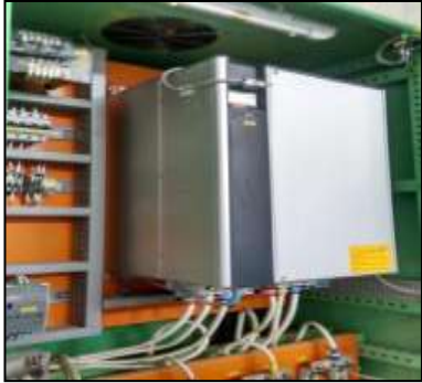
VFD for air compressor
