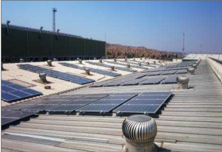
Roof top Solar panels – 250 KW plant
